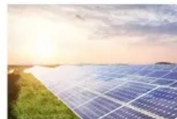
Energy Storage System
